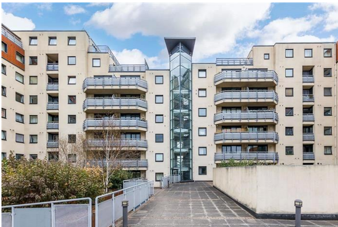
WARDS WHARF APPROACH, PONTOON DOCK, E16 £1,550 PCM
